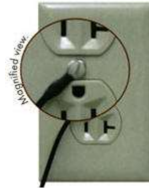
Figure 10, attachment of ring terminal to ground
